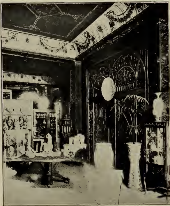
B.—ELEVATOR INCLOSURE, COLUMBUS MEMORIAL BUILDING, CHICAGO, UPPER FLOOR, DIRECT ENTRANCE TO STORE. Wrought Iron, Hammered Leaf Work.
